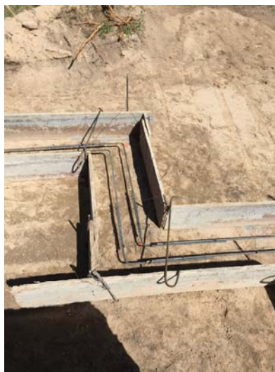
Visual Inspection of footing
