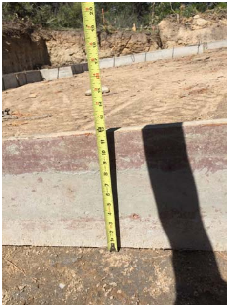
Forms allow 10" depth of placement
