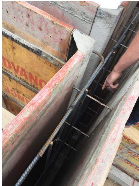
Proper clear cover, vertical, and horizontal rebar spacing (left), proper rebar splice (right)
