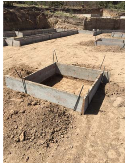
Visual inspection of spread footing
