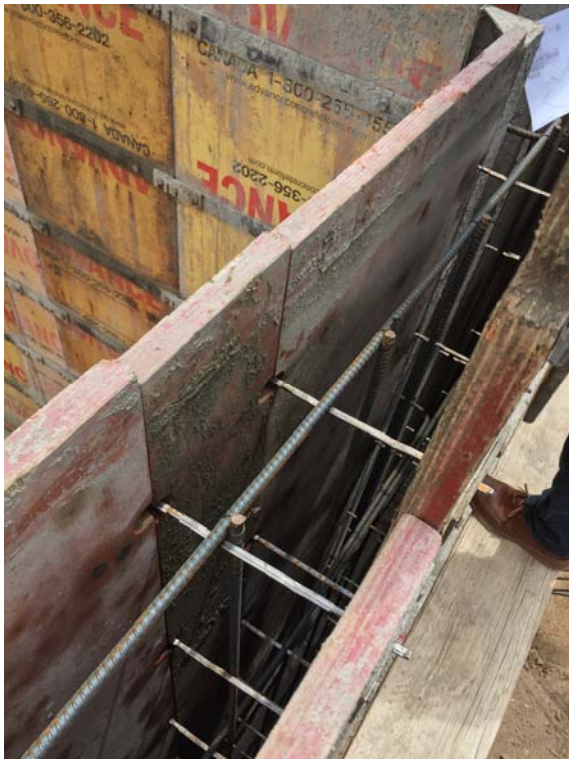
Proper clear cover, vertical, and horizontal rebar spacing (left), proper rebar splice (right)
