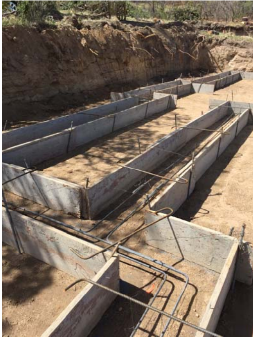
J bars on site
